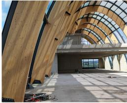
Octatube was asked to develop and build the entire facade for Innovationszentrum Spartherm. The buildin is 40 metres high and consists of over 6500 m2 of glass, with glass panels measuring 5.5 x 2.6 metres. Because of the gradient radius of the facade, many of the glass panels have a different radius. We chose to cold bend a large part of the glass in the work. We developed a special vacuum lifter to handle the large glass panels. This unique vacuum lifter can pick up the large panels,
